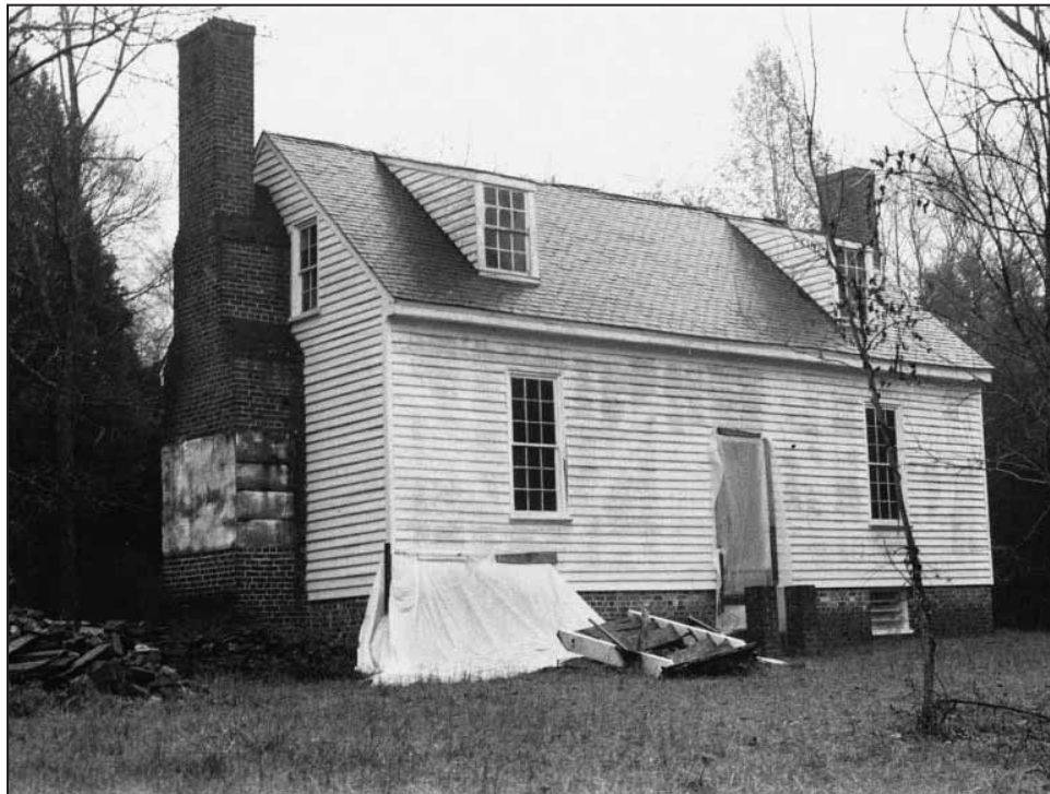
Locust Grove (1997), restoration in process. Courtesy Virginia Department of Historic Resources.
