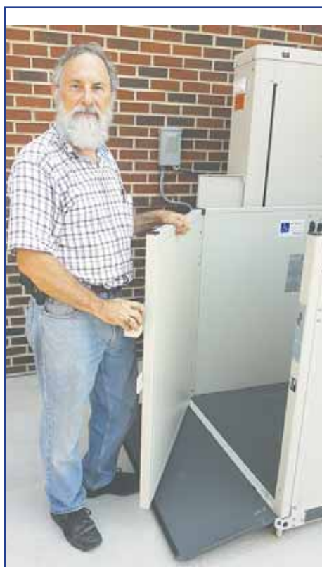
Building committee chairman, Greg Hosaflook, explains how the new wheelchair lift works at Louisa United Methodist Church.
