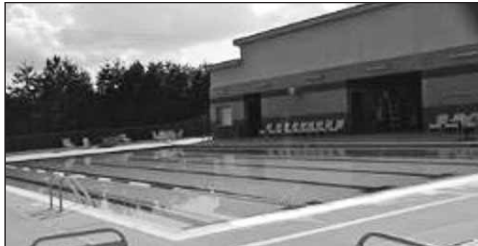
FLCA supports an enclosed structure for the junior Olympic-sized pool at the Betty Queen Intergenerational Center to permit year-round swimming.
