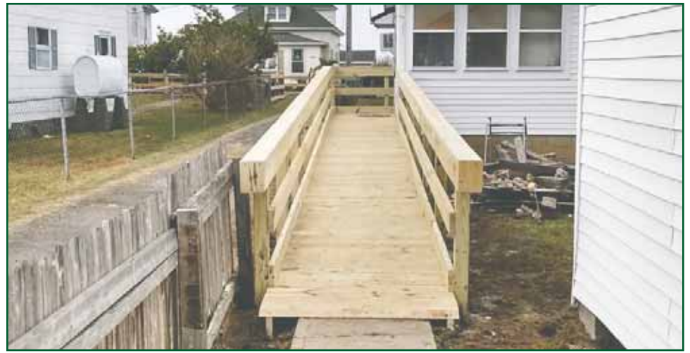
Handicapped ramp addition built by the Tangier Mission Team.
