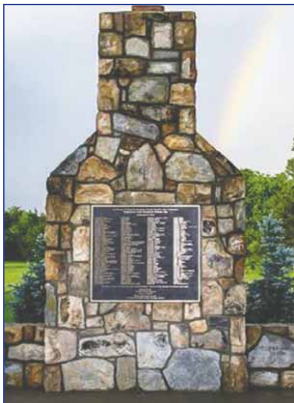
A symbolic chimney erected in Rockingham County as part of the Blue Ridge Heritage Project bears the name of Daniel Shifflett, Sherman Shifflett’s grandfather who was displaced by the creation of the Shenandoah National Park.
