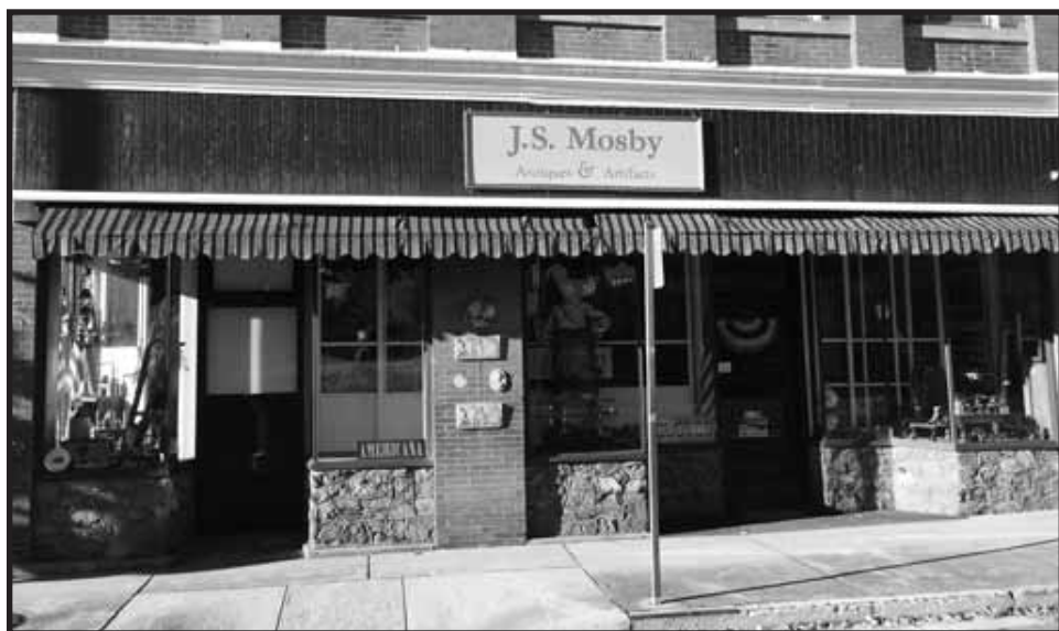
The J.S. Mosby Antiques & Artifacts building can boast that it was the first movie theater in Orange, opening around 1910. The side opening was the concession stand. It was later Grymes Drugstore.
