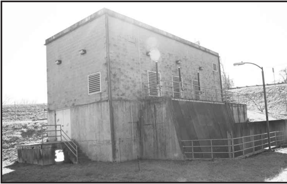
The pumping station. Photos by Ron Smith
