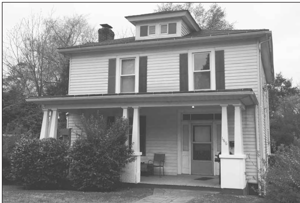
This handsome two-story house is a typical Sears Foursquare design. Photo by Barbara Wimble.
