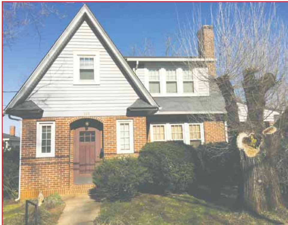
A Sears Lynnhaven house built between 1936-38. Photo by Barbara Wimble.
