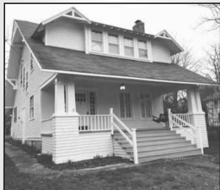
This house in Gordonsville, built circa 1910, is clearly a Sears Arlington design. Photo by Barbara Wimble.
