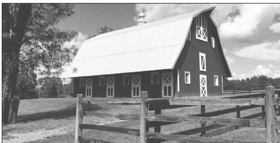
One of the Montpelier Sears barns with a common gambrel-roofed design. Photo by Barbara Wimble.
