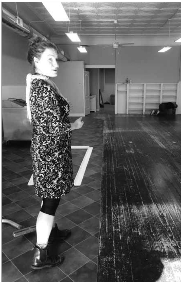
Kristin Hicks stands in the large room that is being developed into a coffee shop. The coffee shop is a building formerly housing The Fabric Hut and Gift Shop.
