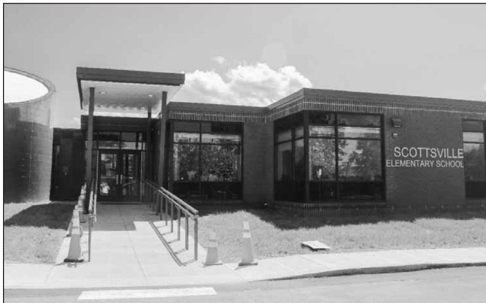
New secure entrance to Scottsville Elementary School. Visitors now must enter the office before being allowed to enter main building. Photo courtesy Albemarle Co. Public Schools
