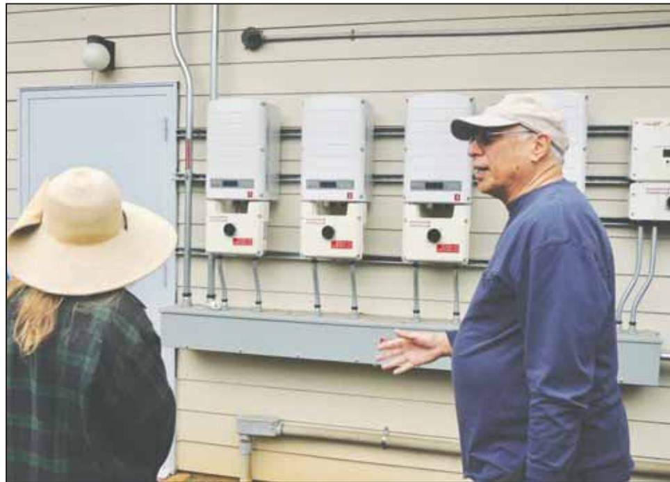
Abeta is shown explaining how the electrical inverters convert the power from the roof array to power that can be transmitted to the electric utility, Central Virginia Electric Cooperative, so that the utility can then turn the meter back per the amount of electricity that they send to CVEC via net metering.
