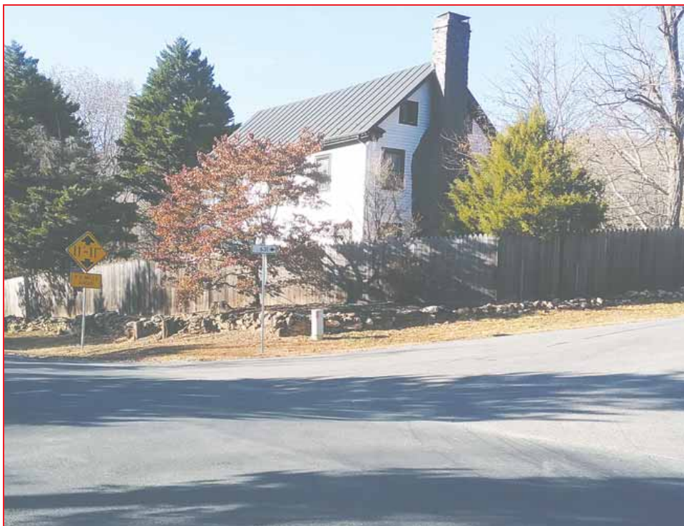
The former Garland's Store on the corner of Plank and Old Lynchburg roads is now a private residence.
