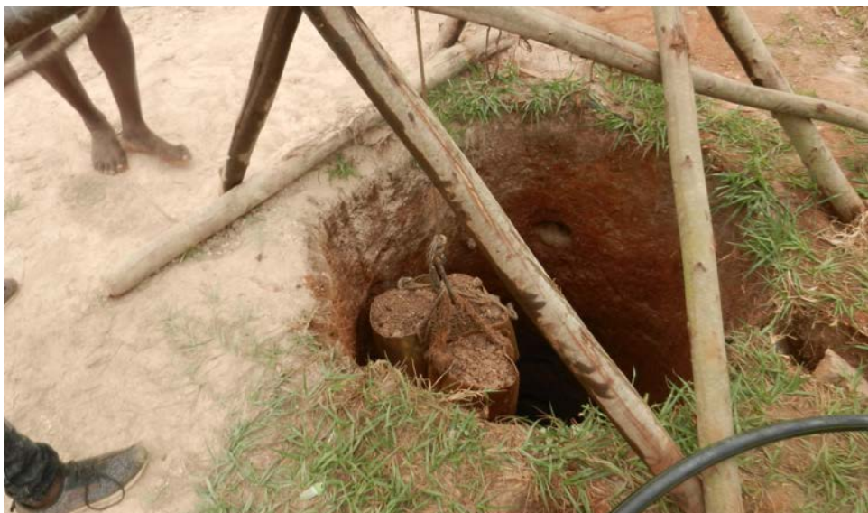
Digging the well by hand.
