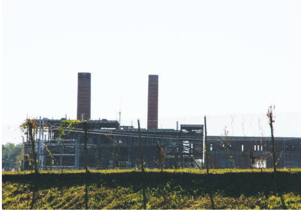
Bremo plant before demolition. Photos by Harvey J. Sorum
