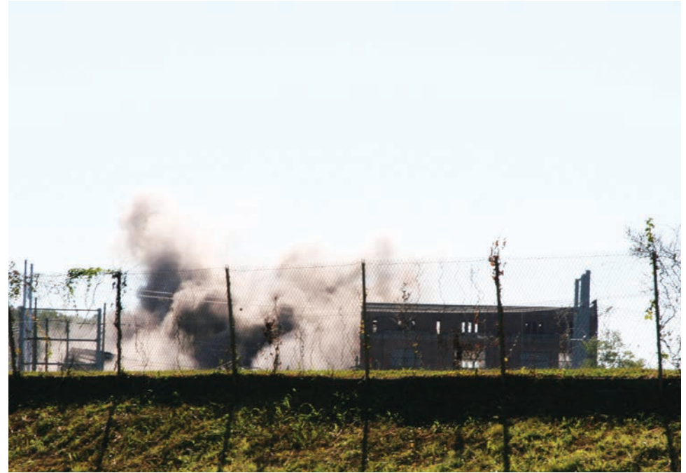
Bremo plant demolished. Photos by Harvey J. Sorum
